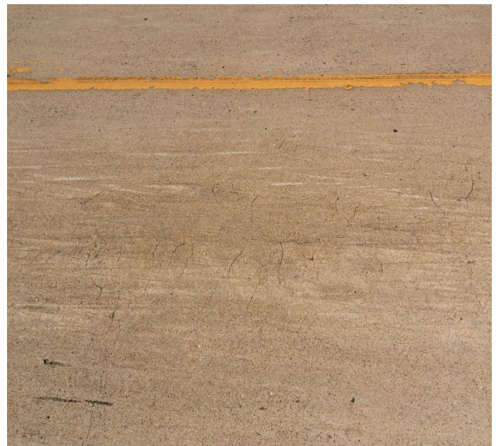
PHOTO 2 Description Span 2 map cracking
