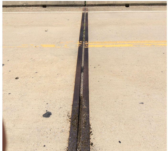
PHOTO 2 Description Bent 3 deck joint seal.
