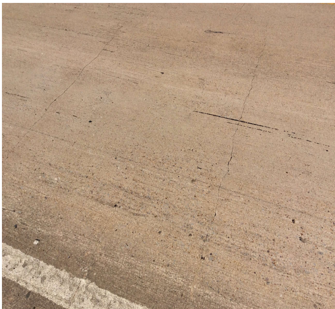
PHOTO 1 Description Sealable deck cracks
