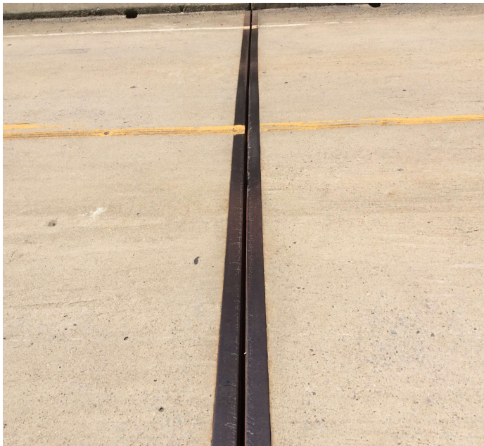
PHOTO 1 Description Missing deck joint seal over Bent 2.
