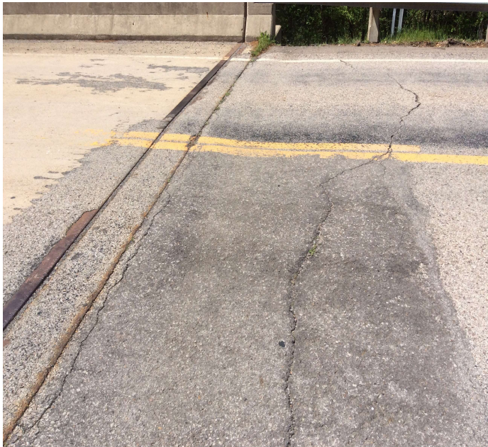
PHOTO 1 Description Asphalt settlement adjacent to Bent 1.
